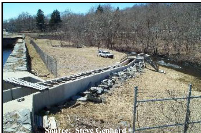
Properly designed Denil fishways will pass fish like those found in the Fox River over dams, but they do nothing to improve habitat or water quality.
